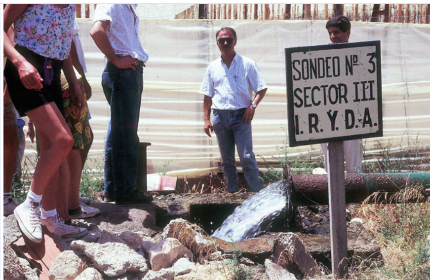
Photo 7.9 One of the boreholes of sector III of Campo de Dalías, producing more than 100 l/s (Photo A. Pulido)
