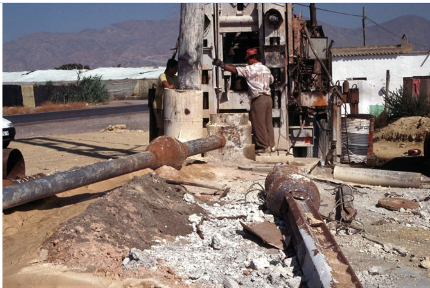
Photo 7.12 Recovering a borehole in the El Ejido area ( Photo A. Pulido )
