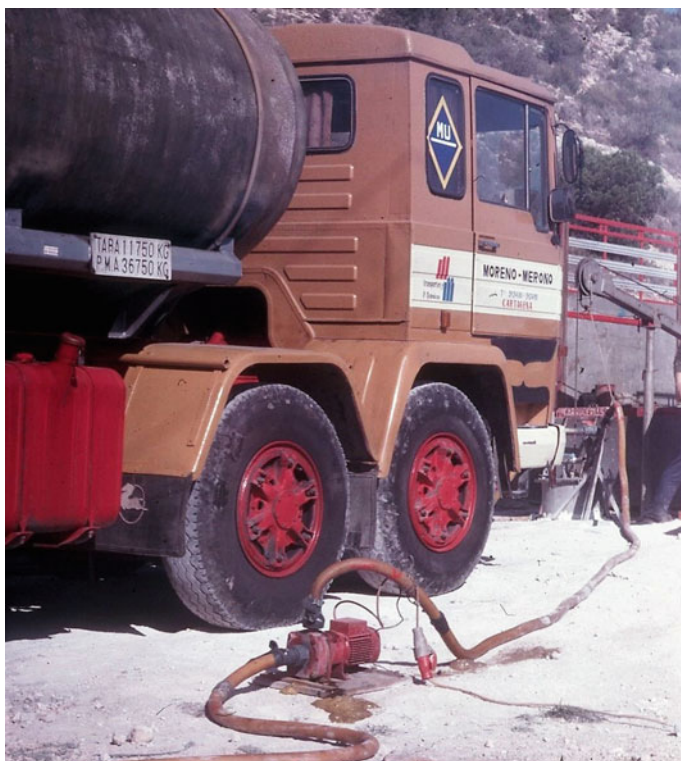
Photo 8.16 Acidification of a borehole in Sierra del Rollo, Aspe (Photo A. Pulido)
