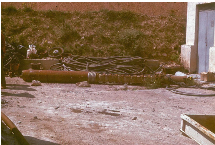
Photo 8.14 Before acidification, it is necessary to extract the pumping equipment; the photo corresponds to a shaft in Aspe (Alicante) sunk by means of explosives (Tolomó sector) (Photo A. Pulido)
