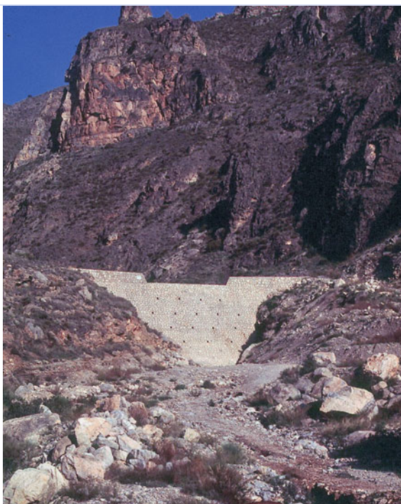
Photo 7.8 One of the numerous hydraulic check dams in this case, which mark the southern edge of the Sierra de Gádor ( Photo A. Pulido )
